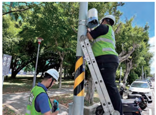
Installation of Micro-sensors
