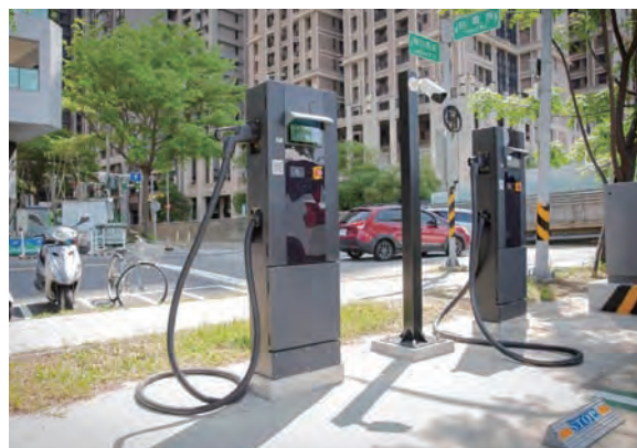
Establishment of Charging Piles
