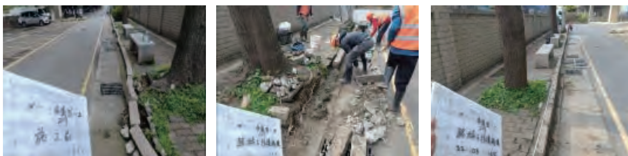
Before construction / During construction / After construction
