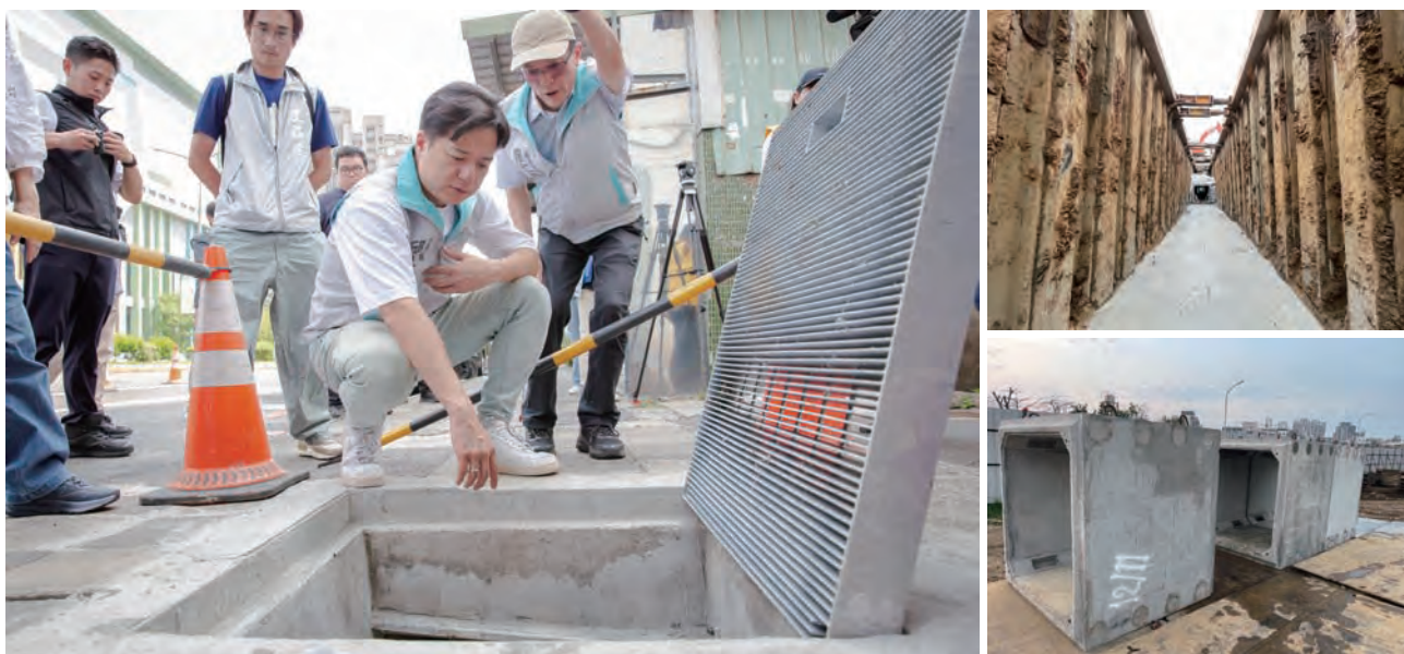
Inspection of the Drainage Improvement Project / Storm Sewer Project
