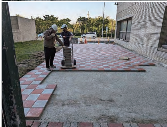
Application of Bricks Made of Incineration Recycled Aggregates
