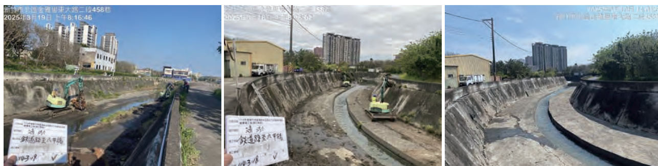
Desilting Operation for Regional Drainage (Dongdapai)
