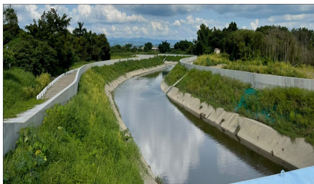
Guizigang Drainage Improvement Project
