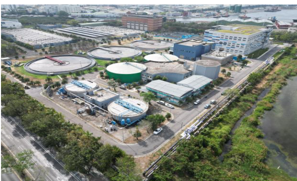
Anping Water Resource Recovery Center and Reclaimed Water Plant
