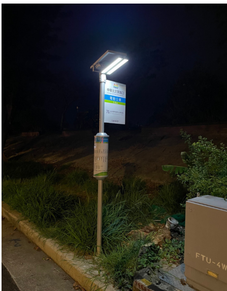
New-Style Solar-Powered Lighting Equipment for Bus Stops
