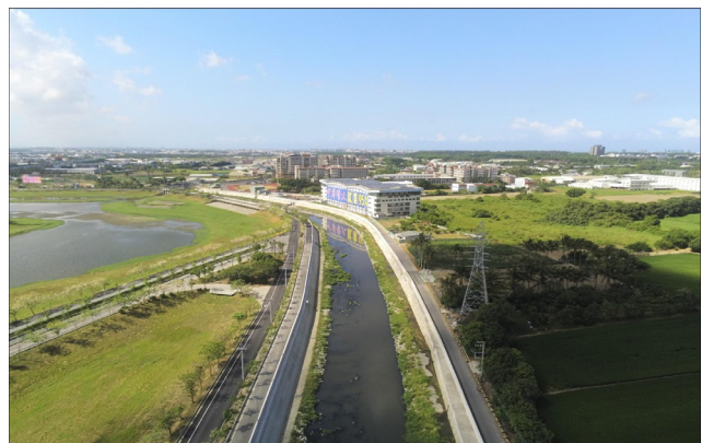
Sanye Creek Drainage System Improvement Project
