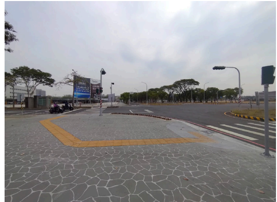
Improvement of Intersections on HSR Boulevard in Guiren District
