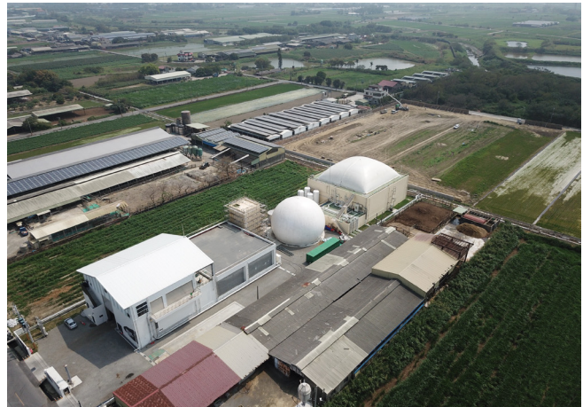
Bawang Village Livestock Manure Resource Recovery Treatment Plant (Phases I)
