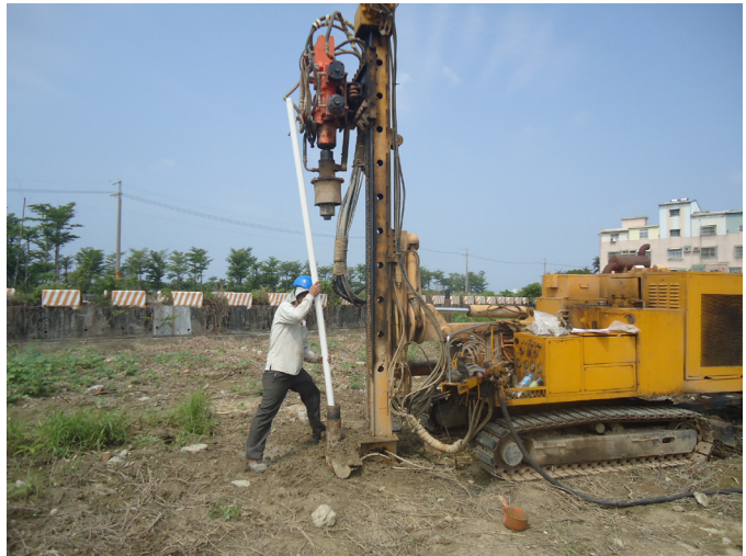
Supplementary Investigation and Installation of New Groundwater Monitoring Wells
