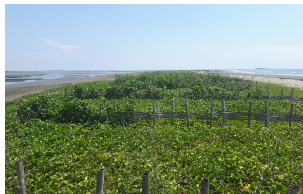
Bamboo Stakes and Sandbag Barriers Against Waves (Left) and Piling with Woven Fences for Vegetation Greening (Right)
