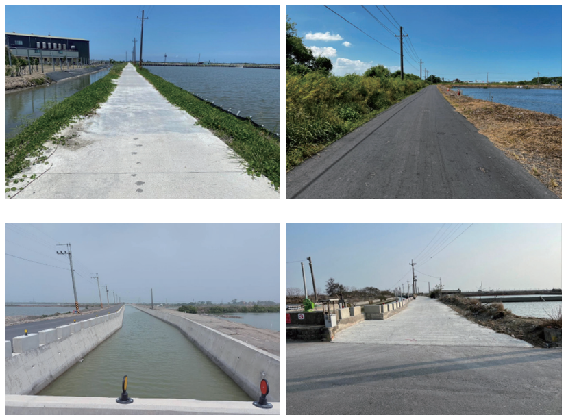
Results of Agricultural and Irrigation Roads Repair and Renovation
