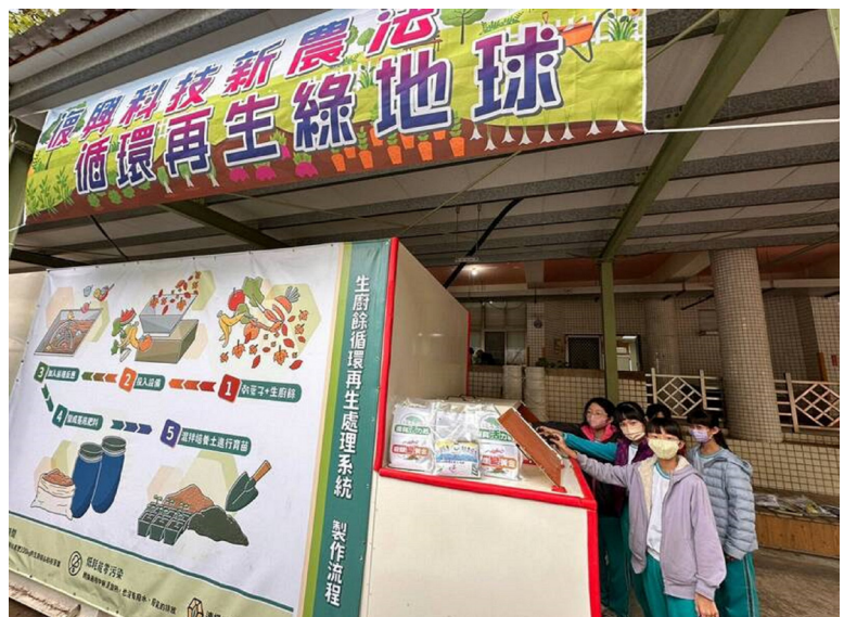
Installation of a Large-Scale Food Waste Processor at Fuxing Elementary School in East District
