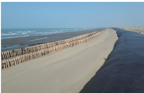
Bamboo Stakes and Sandbag Barriers Against Waves (Left) and Piling with Woven Fences for Vegetation Greening (Right)
