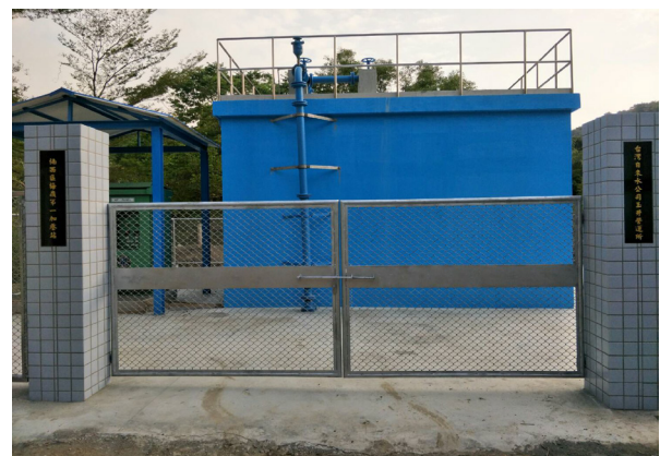
Water Supply to Remote and Rural Areas (Meiling Booster Station)
