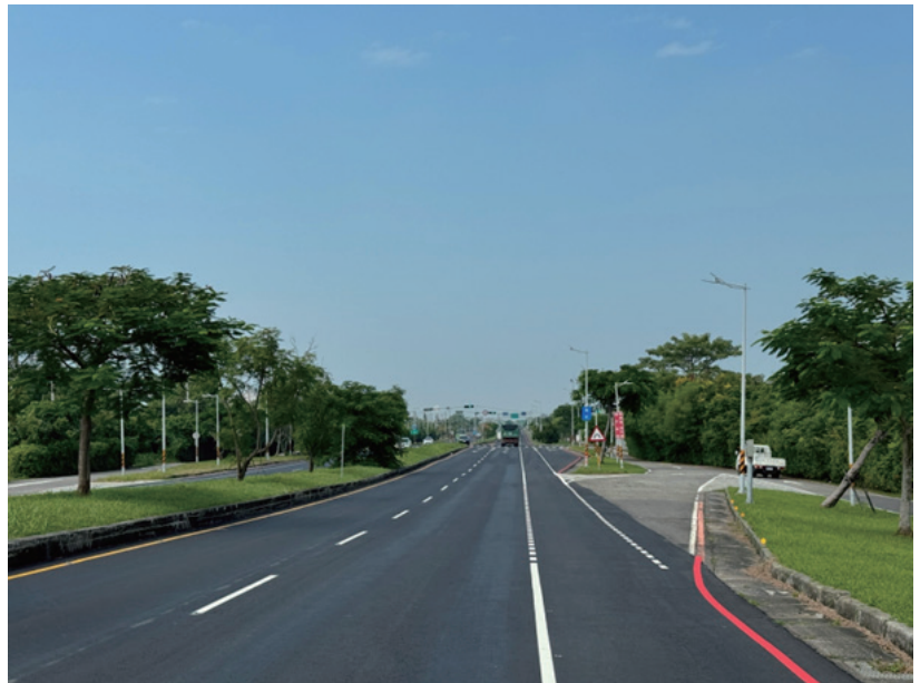
Road Surface Improvement Project on Section 3 of Taijiang Boulevard, Annan District (from Zengwen Creek Drainage to Anming Road)
