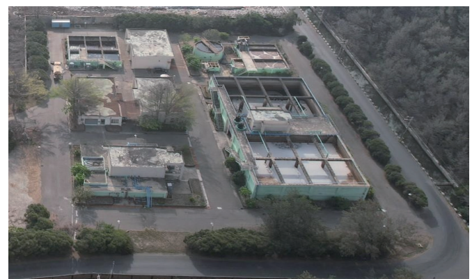
Chengxi Landfill Leachate Treatment Plant
