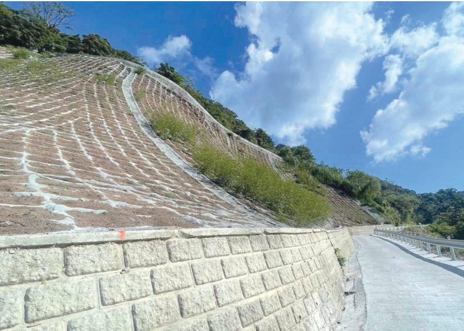
六十石山邊坡工程 Liushishi Mountain Slope Stabilization Project
