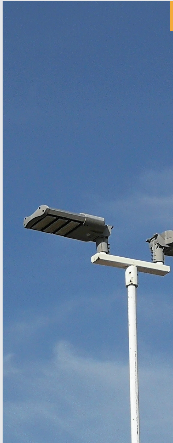
▲ Undergoing the replacement of the LED light
