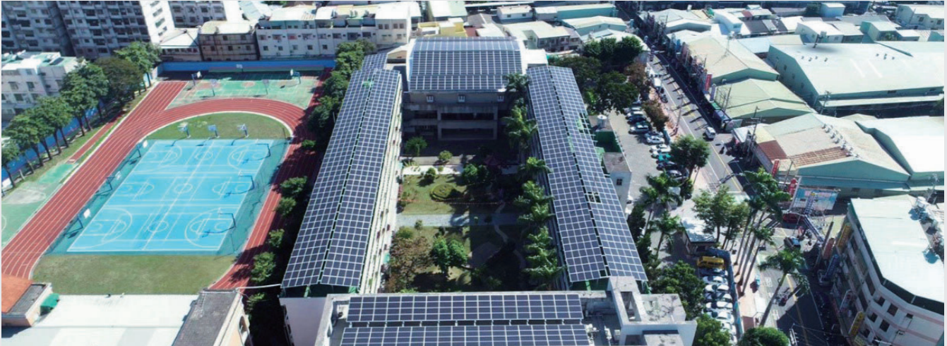
▲ Photoelectric installation on the roof of Taichung City Zhongping Junior High School
