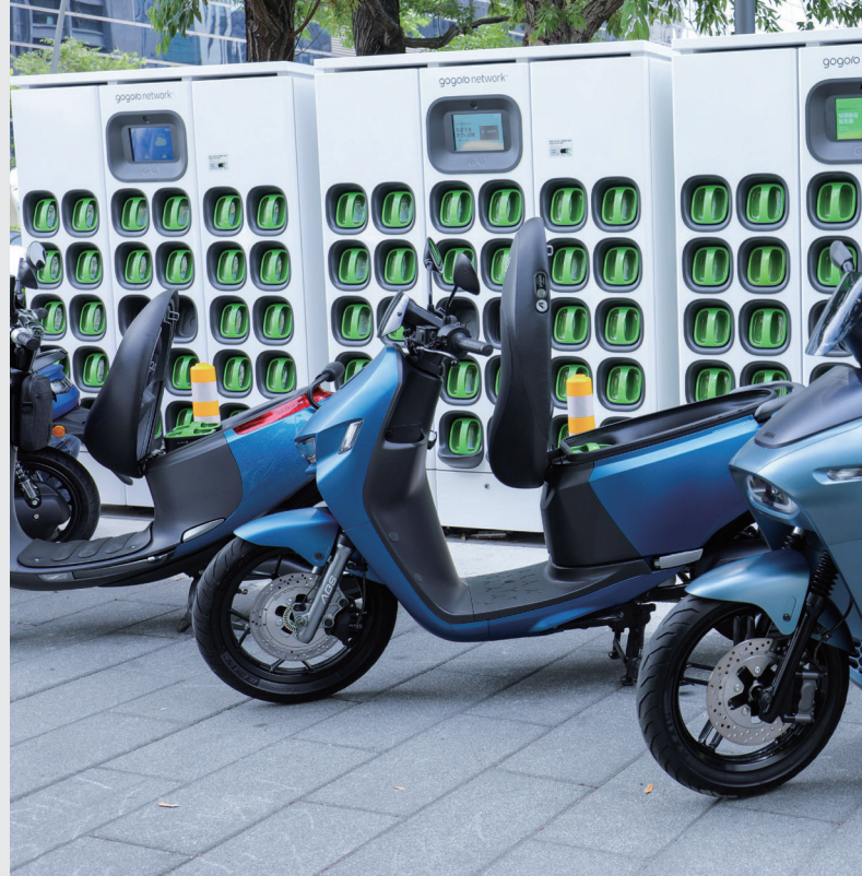
▲ Taichung City GoStation 300th station
