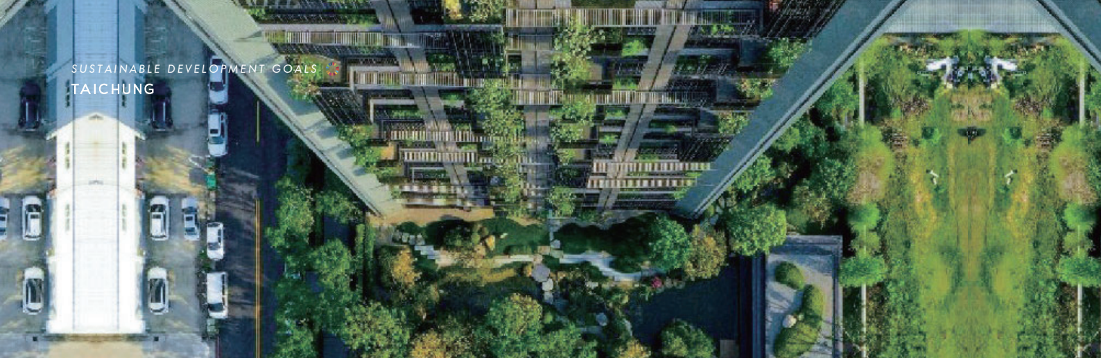
▲ Vertical greening of building façade
