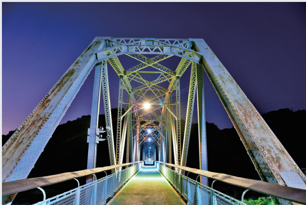
▲ Houfeng railway steel beam bridge
