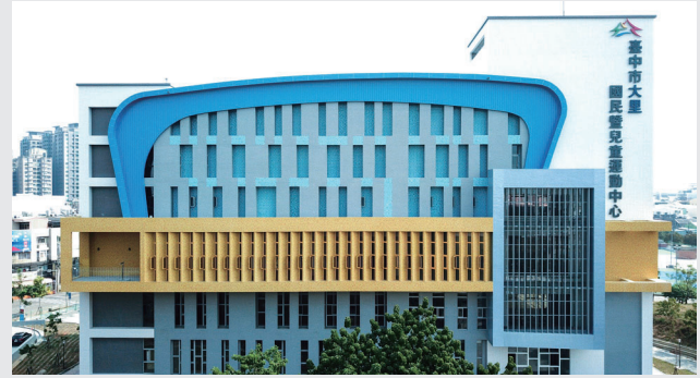
▲ Dali Civil and Sports Center
