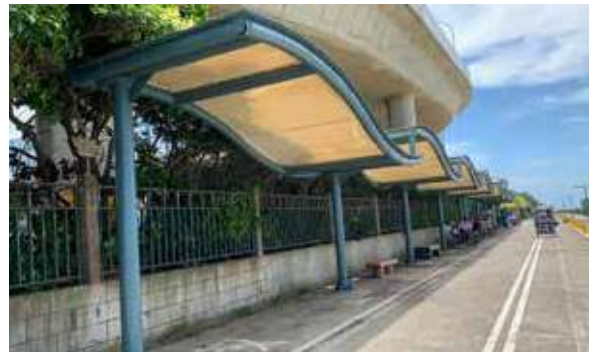
Repairing and varnishing the wooden steps beside the Sea View Park / Wave Pavilion at 17KM, rust removing and repainting
