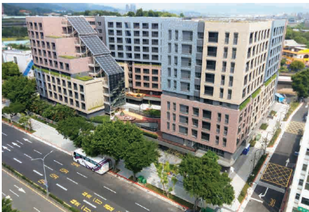
▲ Construct diversified social housing - Minglun Social Housing
