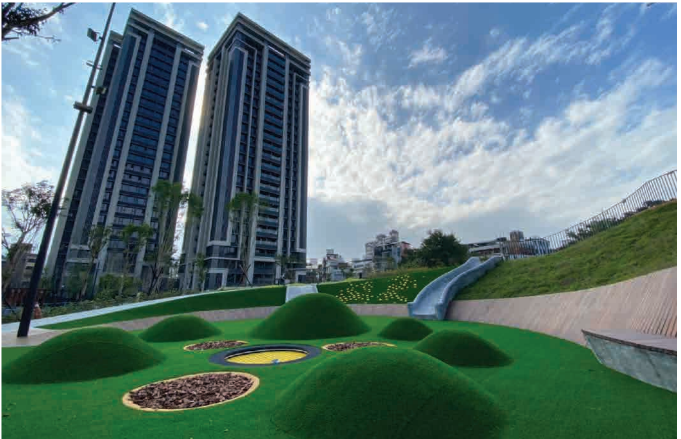
▲ Construction of Xinhai Ecological Park on top of the Military Police Camp Flood Detention Pool on Xinhai Rd.
