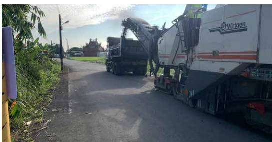
Asphalt removal and replacement
