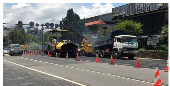
Asphalt removal and replacement
