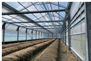
Structural steel frames
