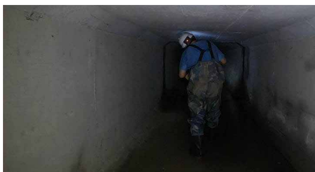
Maintenance of rainwater sewers
