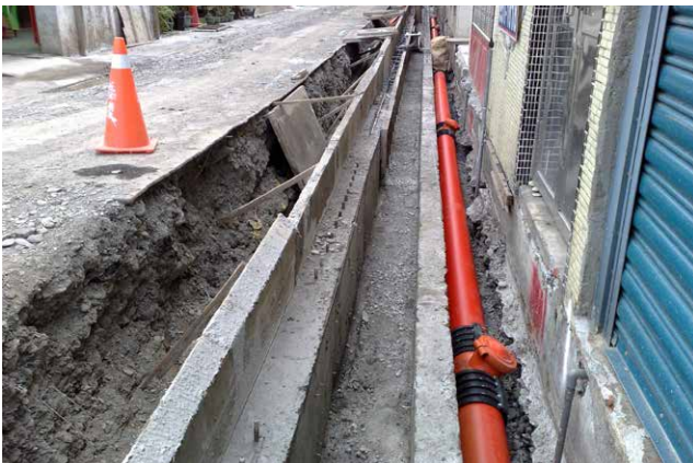
Sanitary sewer system under construction in Dayin Community, Sanxing Township
