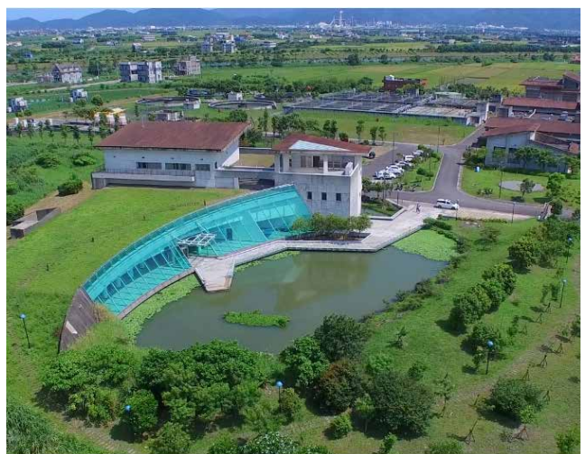
Luodong Water Resources Recycle Center
