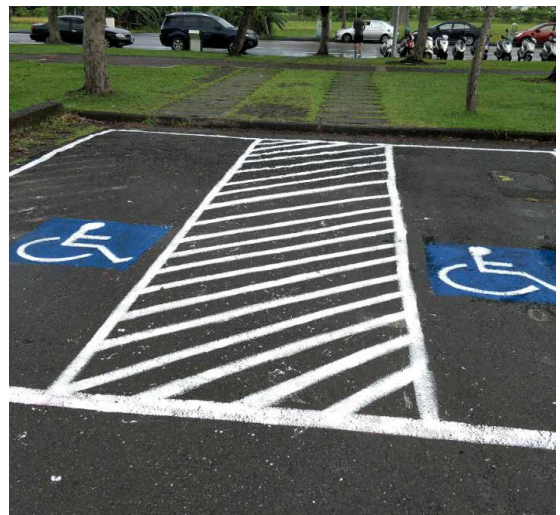
Parking spots with improved accessibility
