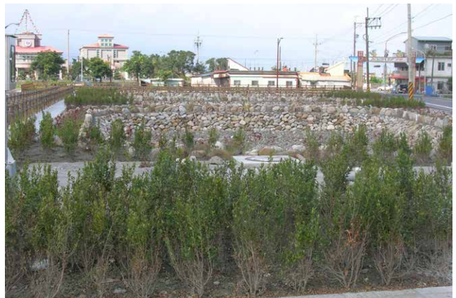
Sewage treatment facility in Dayin Community, Sanxing Township
