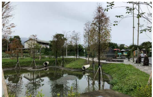
Detention basin facility, Alancheng District, Yuanshan Township
